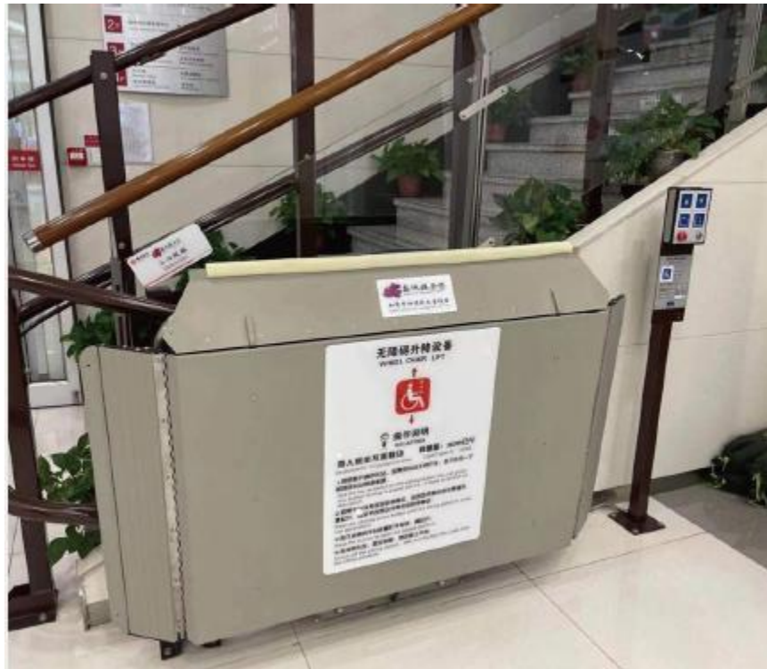
Photo: Construction of barrier-free facilities in outlets
